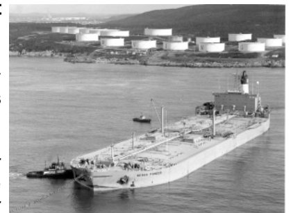
The multi-purpose dock will go in adjacent to the existing Irving Canaport facility at Mispic Point.
