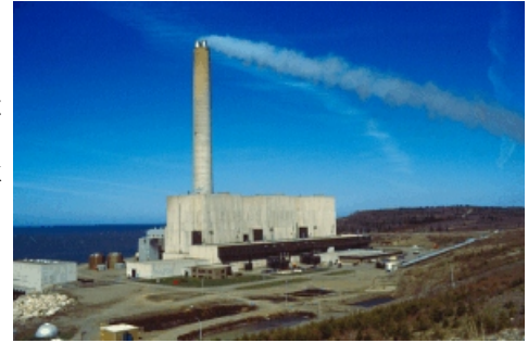
The Coleson Cove Thermal Generating Station on the shores of the Bay of Fundy between Lorneville and the Musquash estuary, a proposed marine protected area. A second huge stack has been erected to the left of the original stack as part of the Orimulsion conversion.
